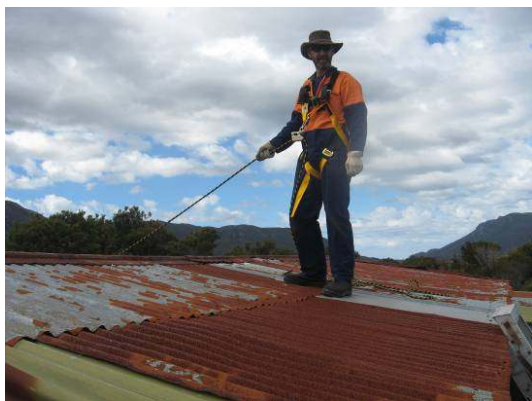
Chris Creese working on the smelter shed roof. Photo: David Butler
