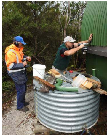
David and Mark installing new guttering, bushwalkers hut. Photo: Ian Marmion
