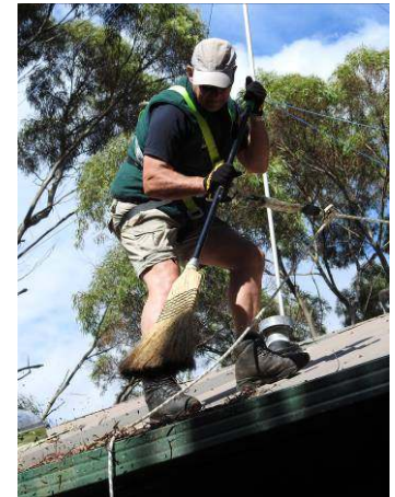
Mark cleaning the PWS Quarters roof and gutter. Photo: Ian Marmion
