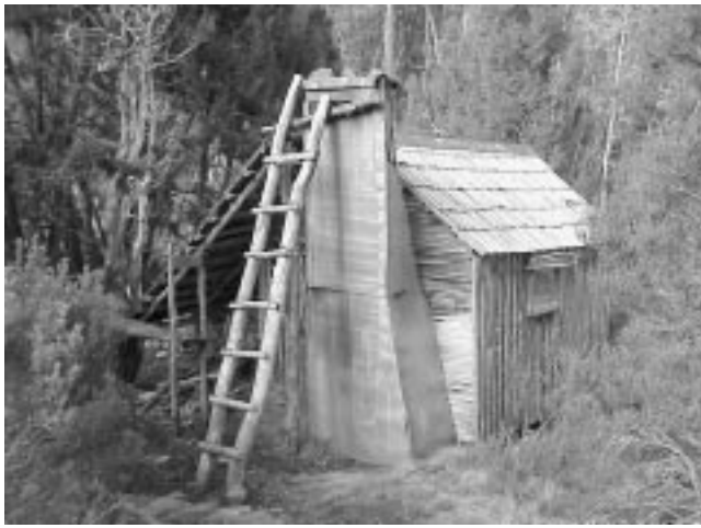
Junction Lake Hut, Walls of Jerusalem NP. Photo PWS.
