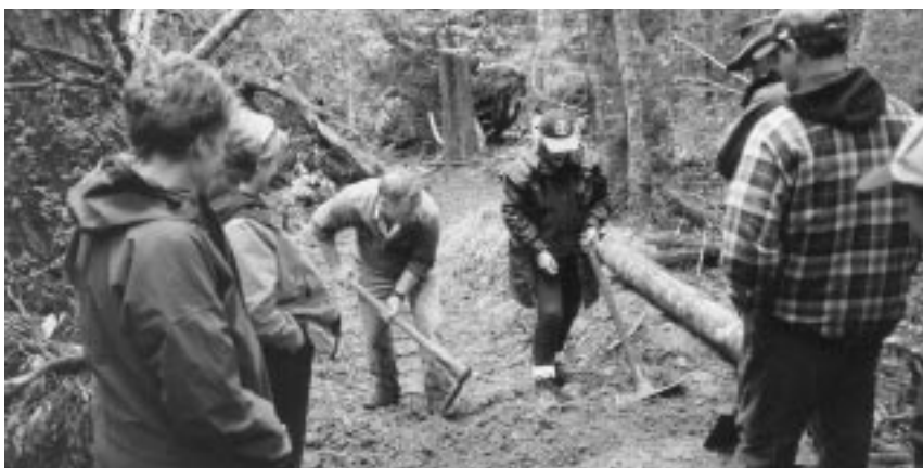
Vonda Sushames shows Dick Dwyer (PWS) how to dig a drainage channel for a waterbar! Photo J Field.
