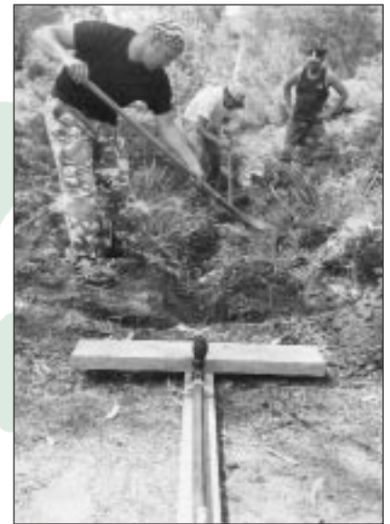
Harry and friends lay a new waterline to Hazards Beach Campsite.
