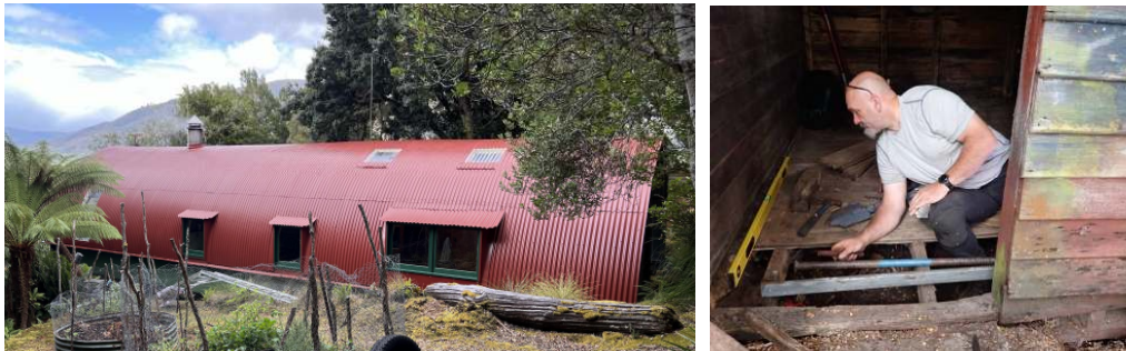
New roof paint at Kings, and shed restitution. Photos: Justin Marshall, Janet Fenton,
